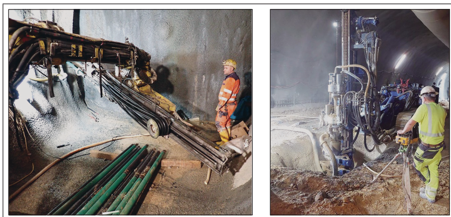
Figure 12. Impression of underground dewatering measures in the Bergzabern tunnel: Left image: Drilling of AT76 drainage boreholes by use of tunnel boomer and rotary percussive drilling equipment in the rescue tunnel. Right image: Drilling of larger diameter vertical drainage well from the crown section of the main tunnel using a HUETTE drill with cased rotary drilling method
