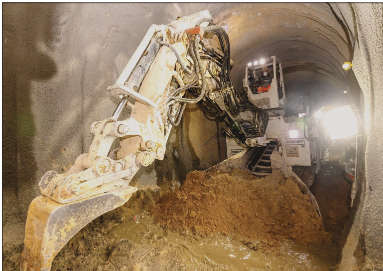
Figure 9. ITC 312 tunnel excavator in the Bad Bergzabern rescue tunnel
