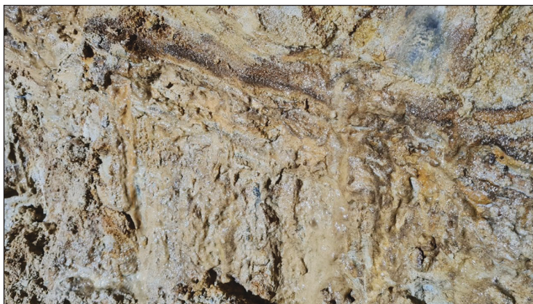
Figure 11. Small-scale flowing of non-cohesive sand (Ground Unit X1) in the face of the rescue tunnel in February 2022
