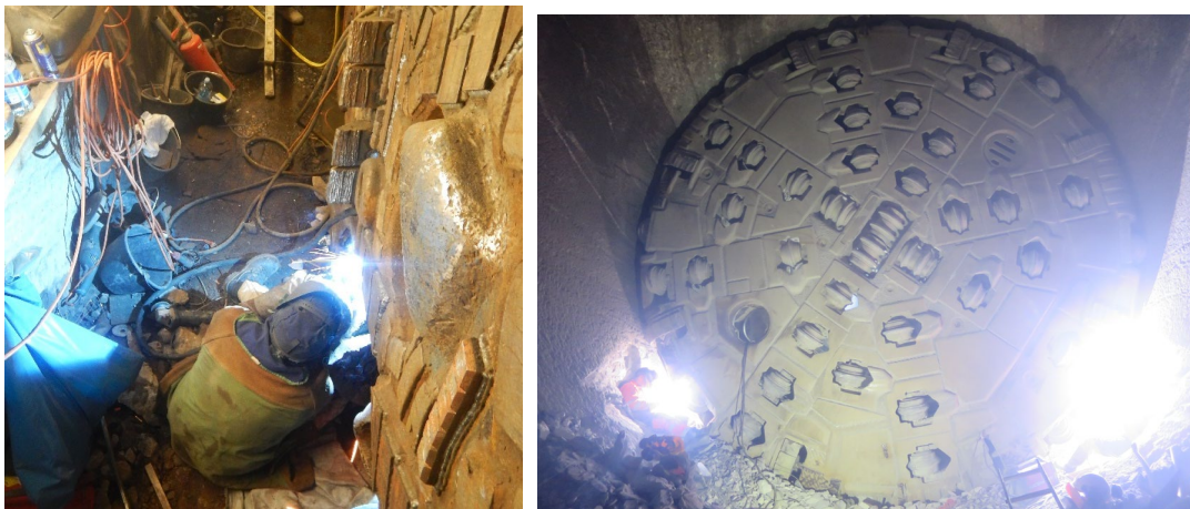
Fig. 1: Underground rehabilitation works in front of a severely worn cutterhead.
