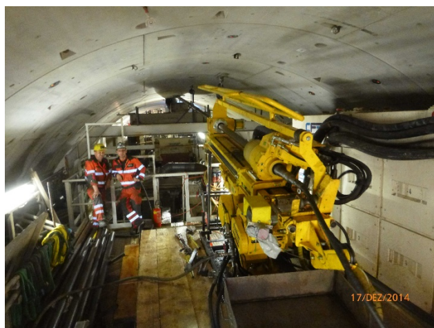
Figure 6. Subhorizontal Core Drilling ahead of the TBM advance from the upper deck of a Ø 10 m doubleshield TBM using an Atlas Copco DIAMEC U6 Drill Rig.
