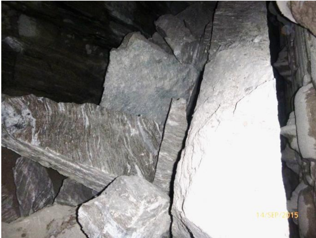
Fig. 3.5: Cubic decimetre to cubic meter large gneiss blocks in front of the cutterhead of a hard rock TBM. Discs and cutterhead can be seen on the right edge of the image (Photo: Plininger).
